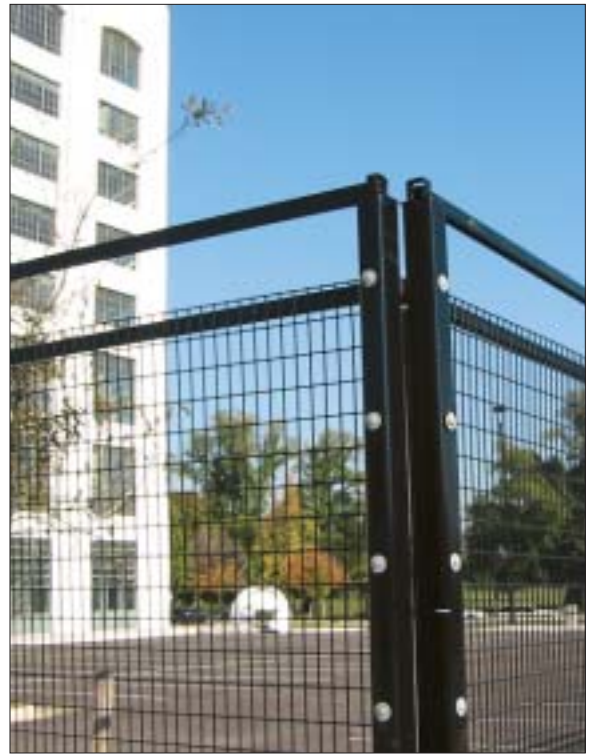
WELDED MESH CORNER POSTS
