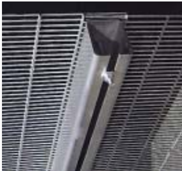
WELDED MESH "C" POST OVERLAP
